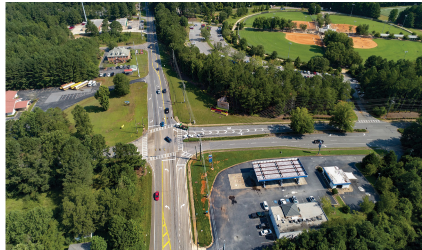
GDOT scheduled to let to construction in January 2025
