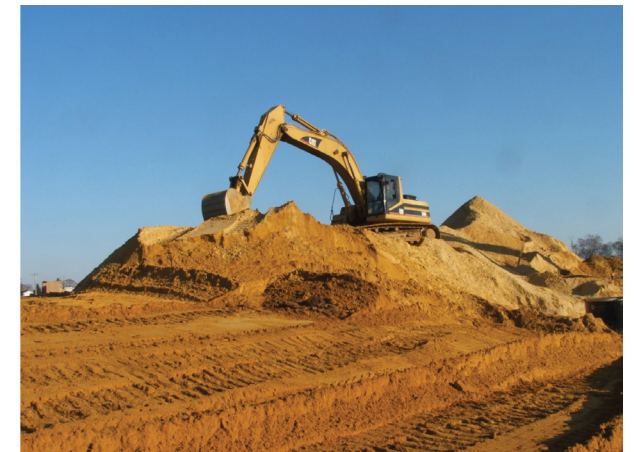
Earthwork for a Subdivision
