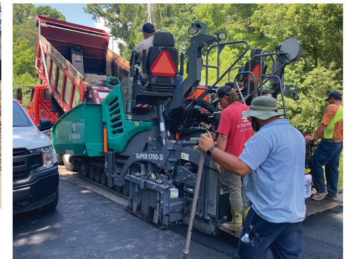
In-House Resurfacing by Public Works
