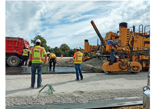
Road Installation Inspection
