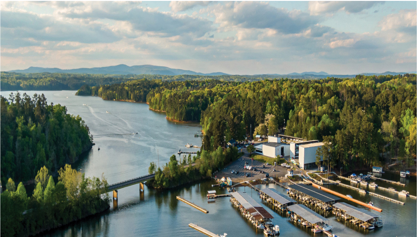
Bells Ferry Road Little River Bridge
