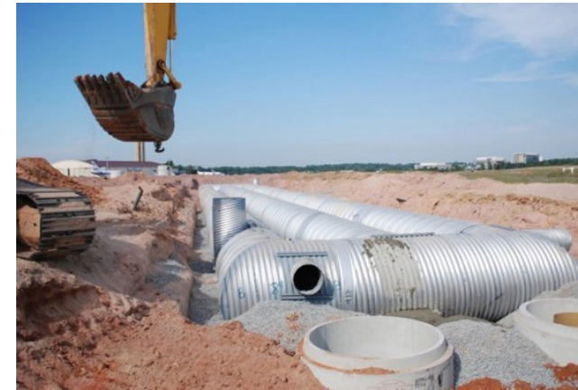
Underground Detention Inspection
